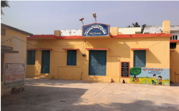
Gorlivanipalem Zilla Panchayat Office
